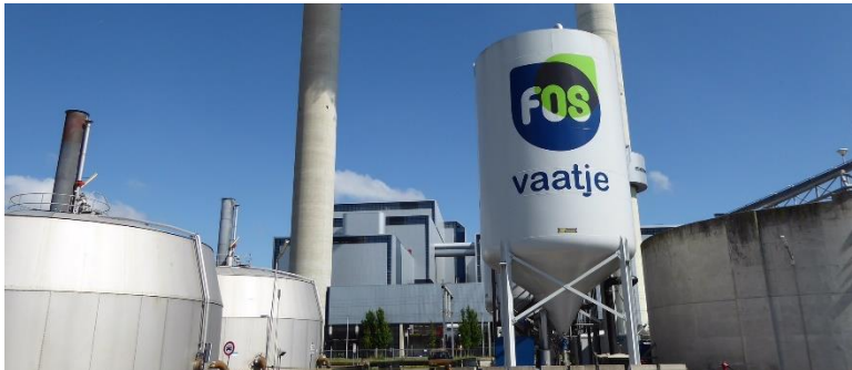
Recovery of phosphate from waste water 700 ton/yr struvite in 2027
